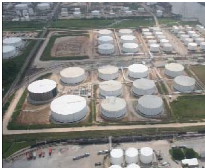
Kinder Morgan has almost 20 million barrels of storage capacity at its two Houston terminals. More than 1 million barrels of product is moved each day. The Galena Park terminal, where the biodiesel storage is located, has 4.5 million barrels of storage.
